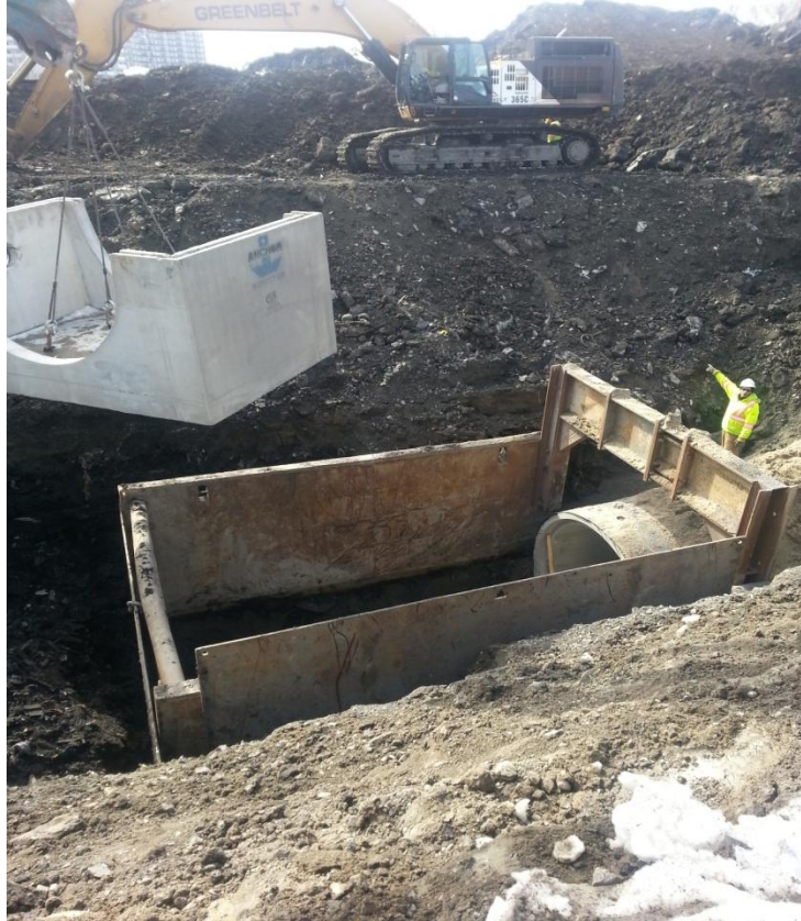
Large diameter Storm Sewer installation – April 8, 2015
