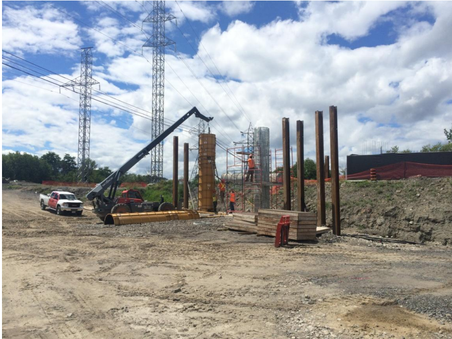
Construction of Riverside structure pier columns.
