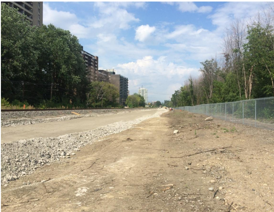
Construction of VIA rail diversion embankment.
