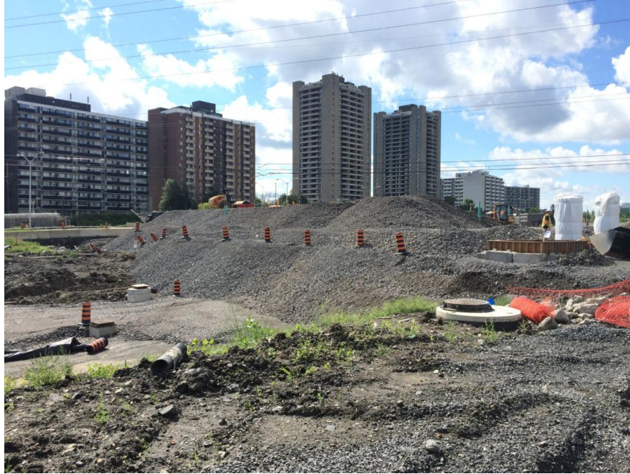
Surcharge for Riverside structure deck falsework.
