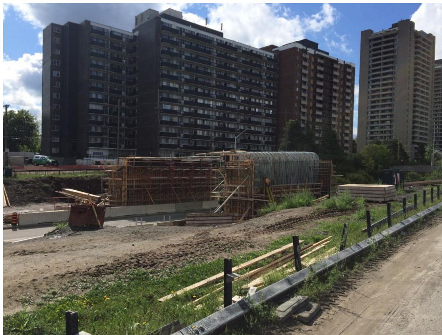
Surcharge for Riverside structure deck falsework.
