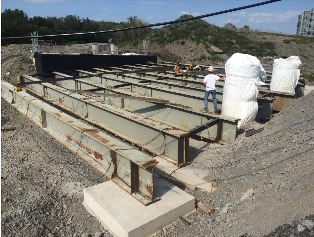
Support Girders for Riverside structure west span falsework.
