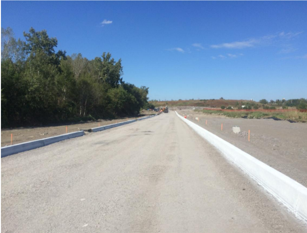
Road construction of Hospital Link, west of Riverside Drive.
