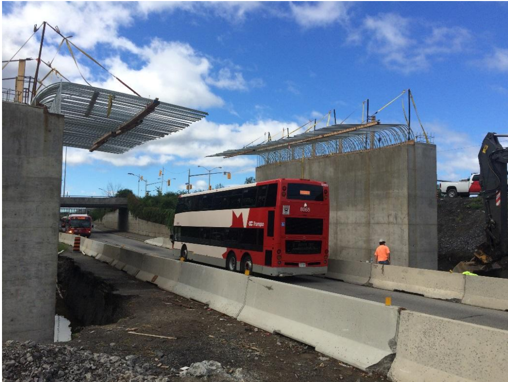
Transitway abutments completed.
