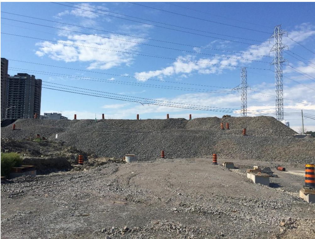
Surcharge placed for the east and center span of the Riverside structure, in preparation for falsework.
