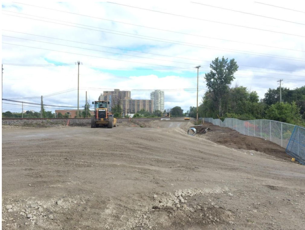
Construction of VIA rail diversion embankment.
