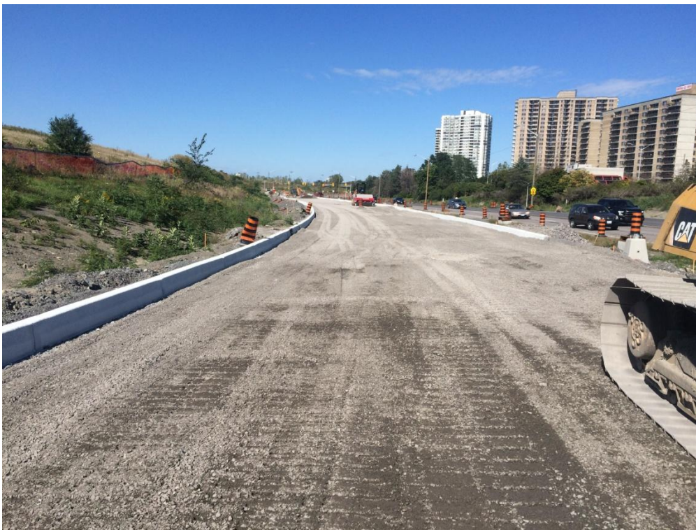
Road construction of Realigned Riverside, between Hincks Lane and Frobisher Lane.
